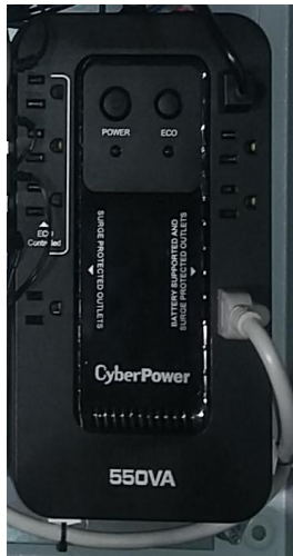
UPS (Uninterruptible Power Supply)
